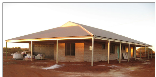
Newman Airport House
