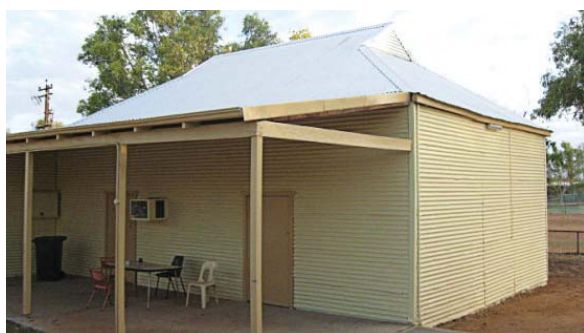
Nullagine – Gallop Hall – New roof and kitchen
