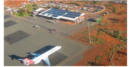
Solar panel on Airport Terminal Roof
