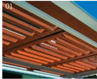
01 Use of horizontal louvers to screen buildings from afternoon sun
