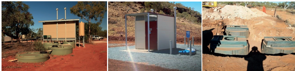
MRWA sites with a sophisticated hybrid system (left) and MRWA Special, under construction with extra tank for sullage (centre & right).
