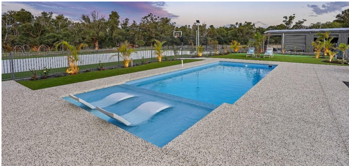
Figure 39 Example swimming pool installation for Nullagine
